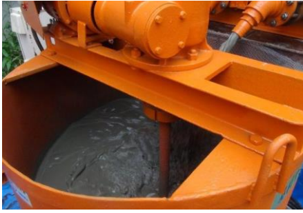
(a)基材練混ぜ状況
